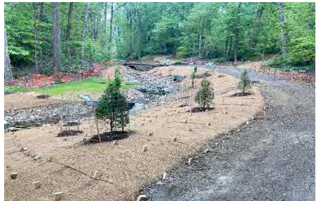
The after picture, above, shows the new channel with step pools to manage and direct the energy of the flow.
