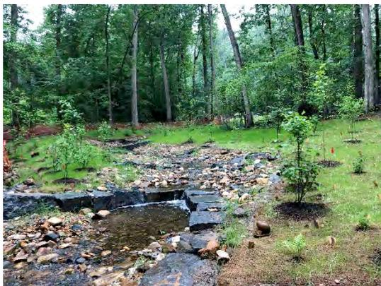
*The picture above shows the new channel with step pools to manage and direct the energy of the flow.*
